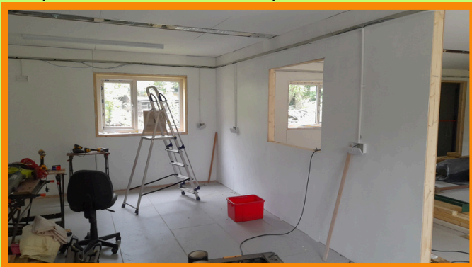
The partition wall - built, painted and wired
