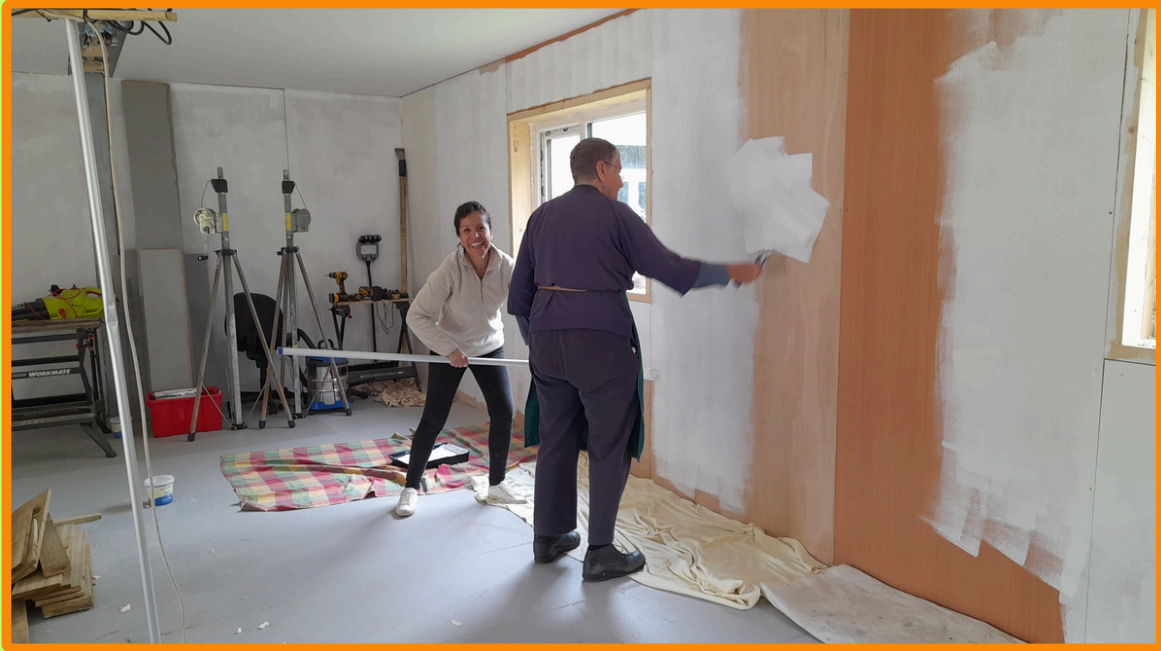
Gaby and Rose just finishing the first coat
